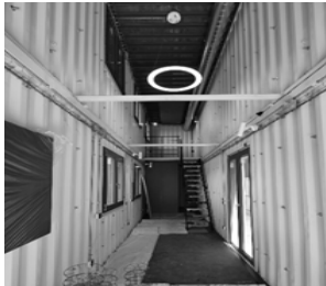
Double-height floor made by overlapping an overturned HC on a base HC, demonstrating the high flexibility and spatial and structural potentiality of the system (it is the first example of this use of HC)
