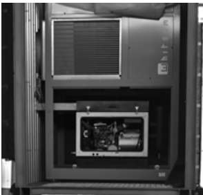
The energy core of the system: an integrated skid for energy and environmental management. Low voltage heat pump integrated to a bio-ethanol co-generator, automatically regulated
